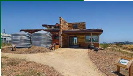
EcoCenter at Heron's Head Park with stormwater collection cisterns
